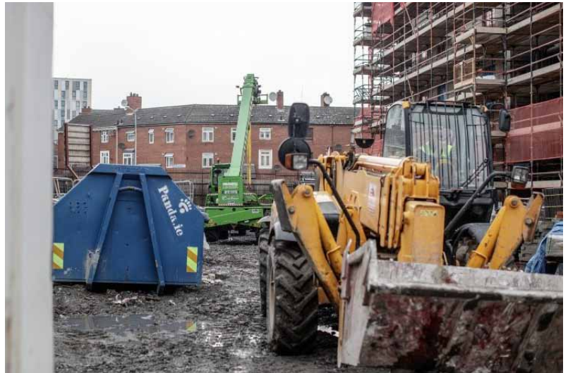
Construction taking place at the Docks and St. Mary's Mansions.
