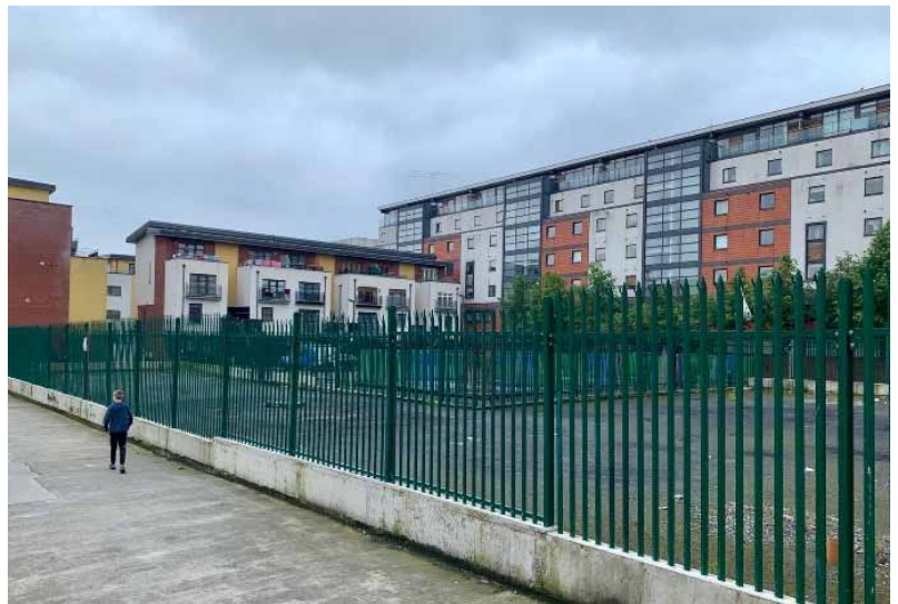
Housing development will commence on this site in the NEIC in Q4 2019.
