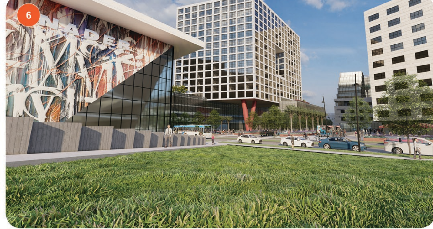
THE BERM AT THE SCULPTURAL PARK, SET ATOP THE RETAIL STRUCTURE ALONG THE SOUTHBOUND PLATFORM, PROVIDES FLEXIBLE OPEN SPACE FOR PICNICS, CONCERTS, AND ART EVENTS THAT SPILL OUT FROM THE NADER ART MUSEUM.
