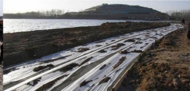
Concrete mixed w/ coal ash as road base material
