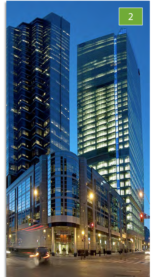
155 Wellington St. W. RBC Centre (1,200,000 sf) 100% Leased (2009) Cadillac Fairview
