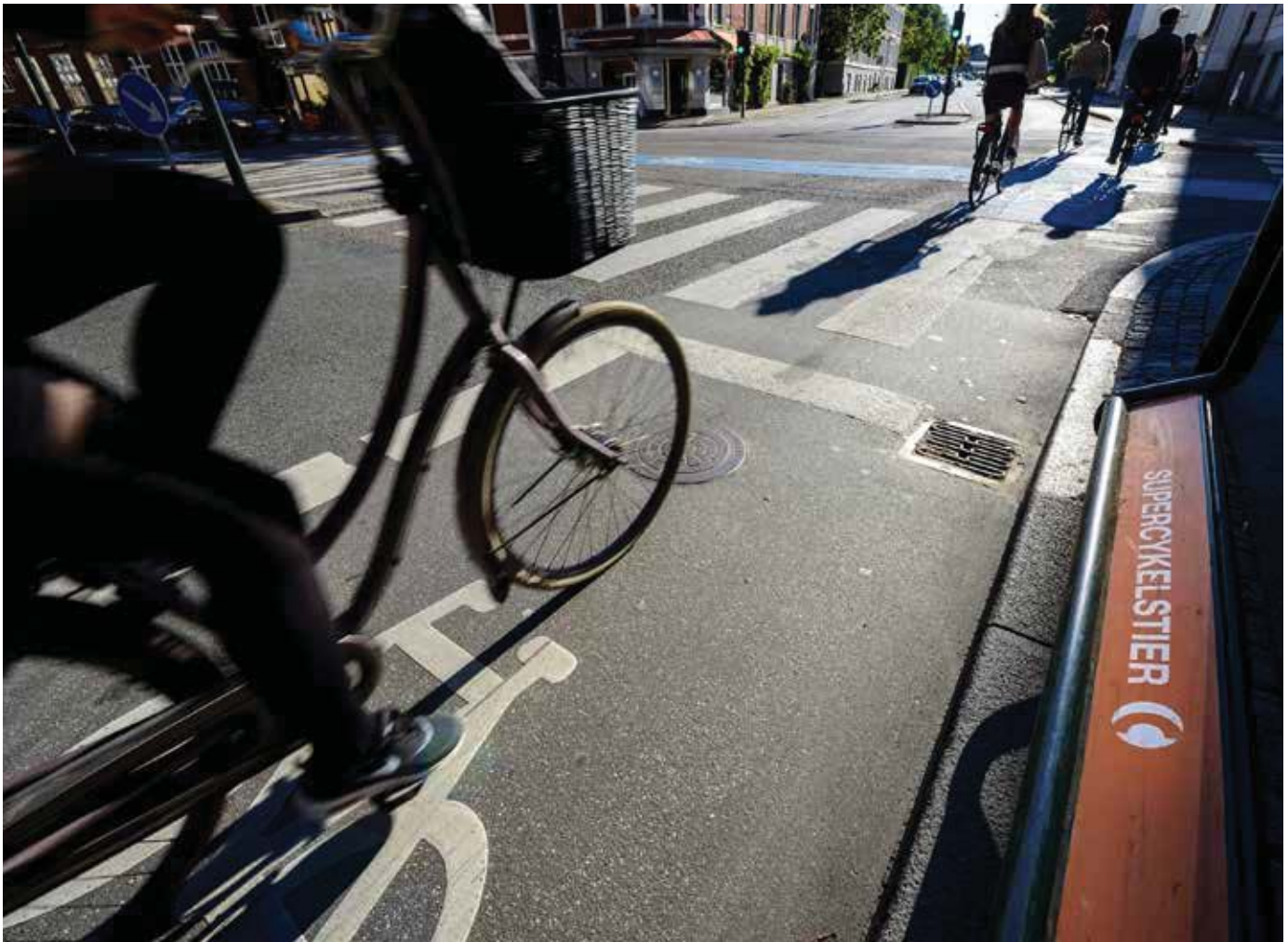
Footrests allow users of the cycle superhighways to stop at red lights without having to get off their bikes. (Copenhagen Cycle Superhighways)
