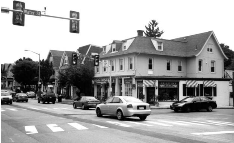
The panel has identified several intersections along Lancaster Avenue that could be upgraded to improve traffic flow.
