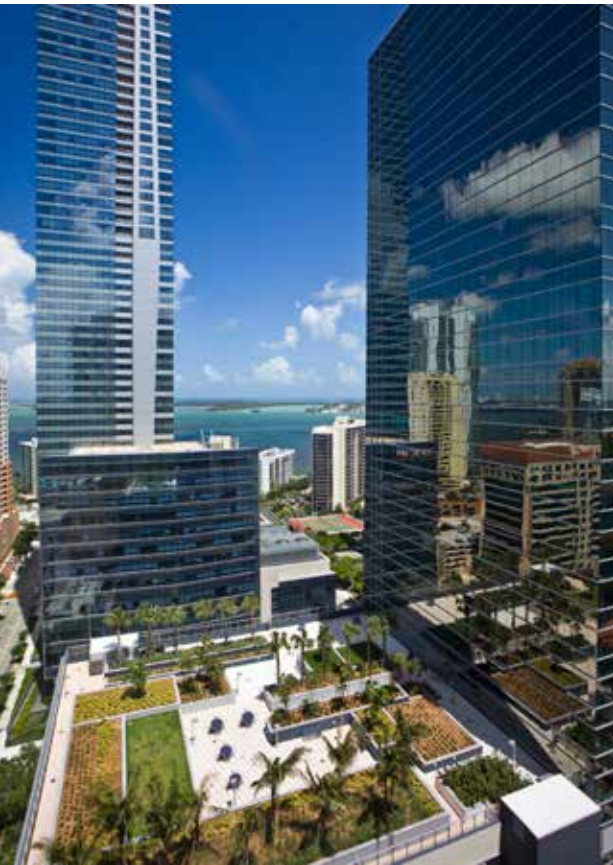
A view of the green roof at 1450 Brickell, Miami, Florida, which was profiled in Returns on Resilience: The Business Case.
