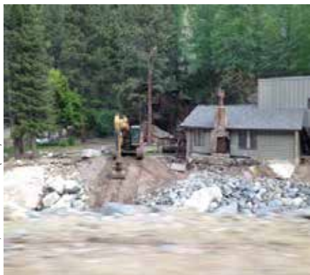
Damages observed after the 2013 floods in northern Colorado.
