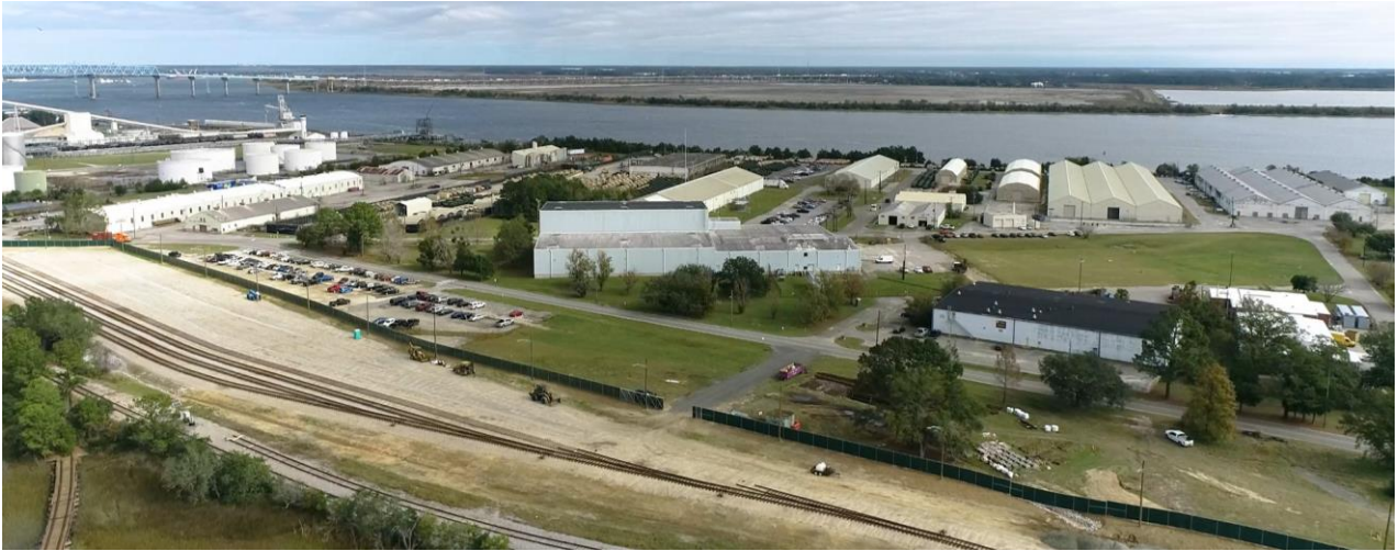
Figure 13. A view of the site looking toward the east across the rail line and the Cooper River. (ULI/Karl Brenkert)
