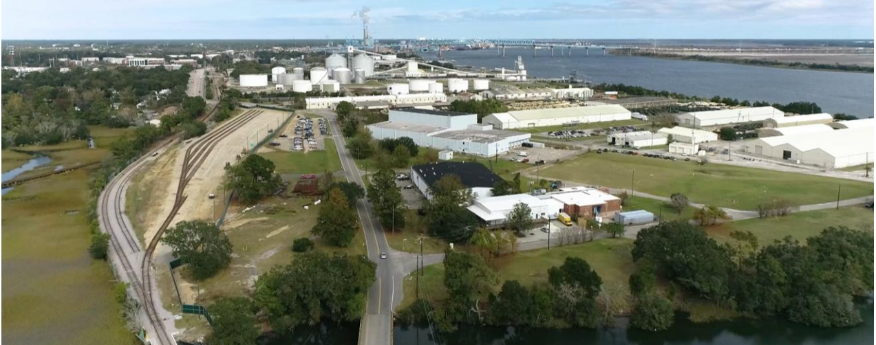
Figure 12. A view of the site looking toward the northeast. (ULI/Karl Brenkert)
