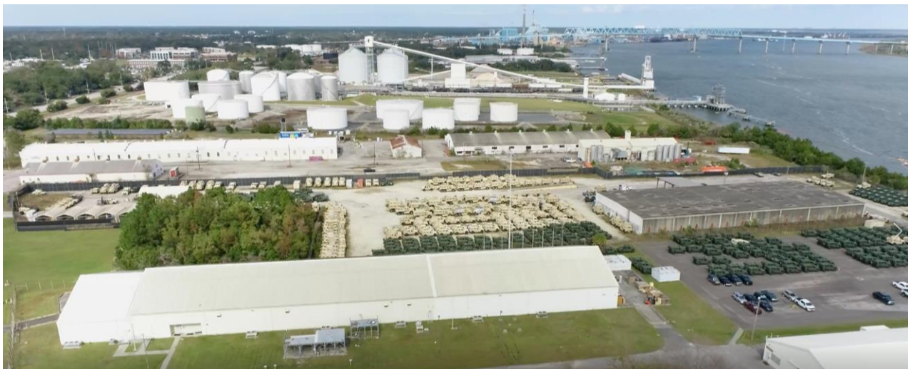
Figure 8. A view from the competition site looking north toward Odfjell Terminals Charleston (OTC) and the Don N. Holt Bridge over the Cooper River. (ULI/Karl Brenkert)
